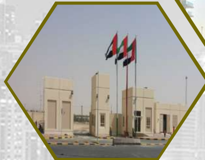
Administration Complex - Abu Dhabi
