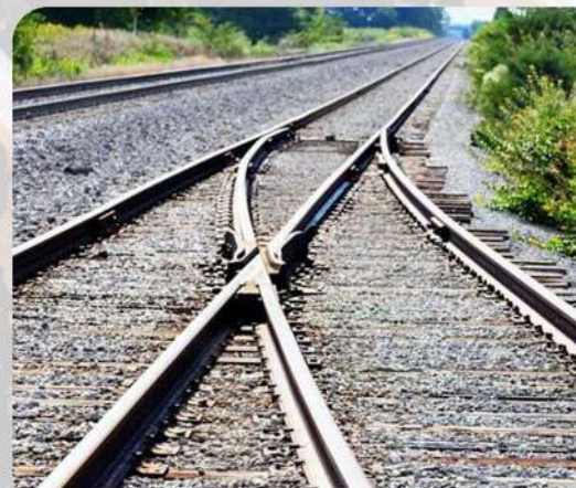
Dualization of Railway Track from Khanewal to Raiwind Length 256 Km
