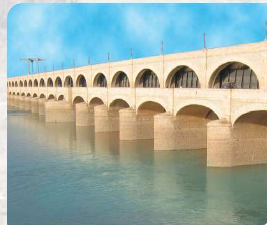
Rehabilitation of Sukkur Barrage
