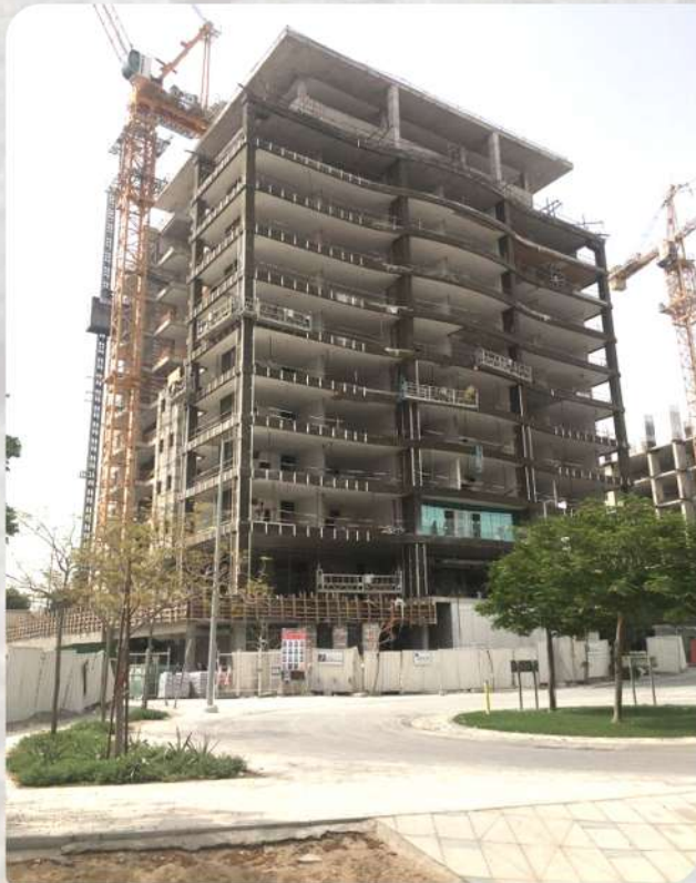
Commercial Building 3B + G + 10 + Al - Raha Beach - Abu Dhabi (P-17)
