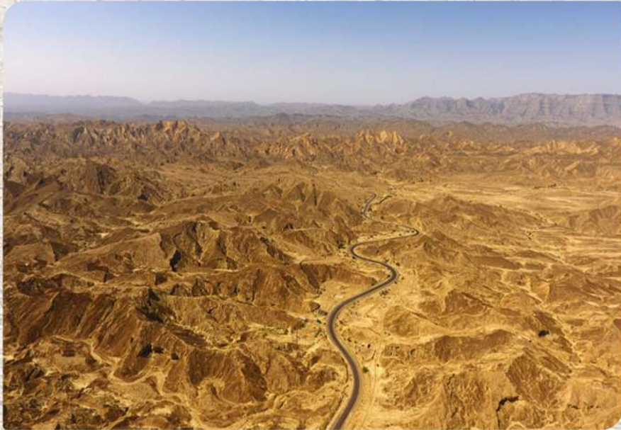
Makran Coastal Highway (N-10)
