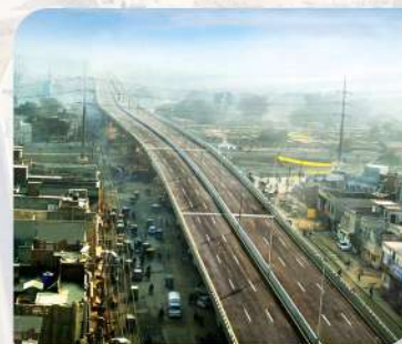
Shalimar Flyover – Lahore
