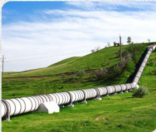
White Oil Pipeline Machike - Thalian - Taru Jabba
