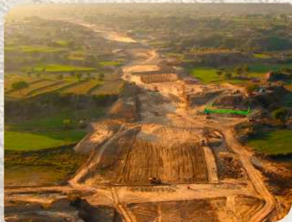
Rawalpindi Ring Road
