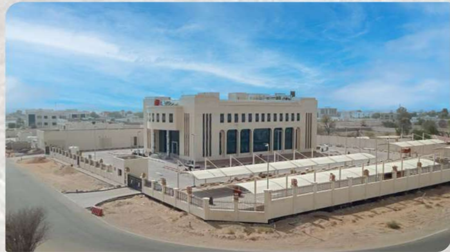
Civil Defence Complex, Falaj - Al- Mualla Umm Al Quwien (P-19)
