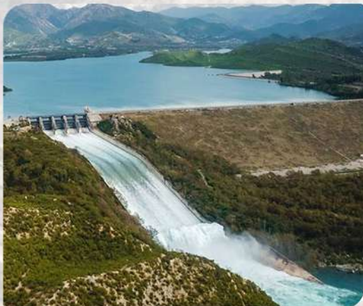
Khanpur Dam - Khyber Pakhtunkhwa
