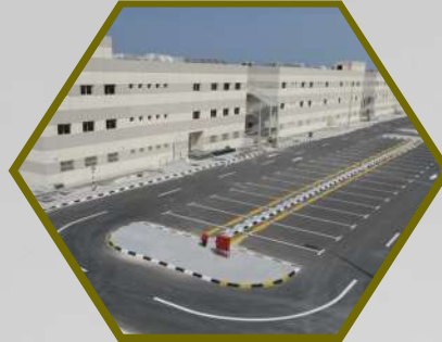
Residential Complex - Abu Dhabi
