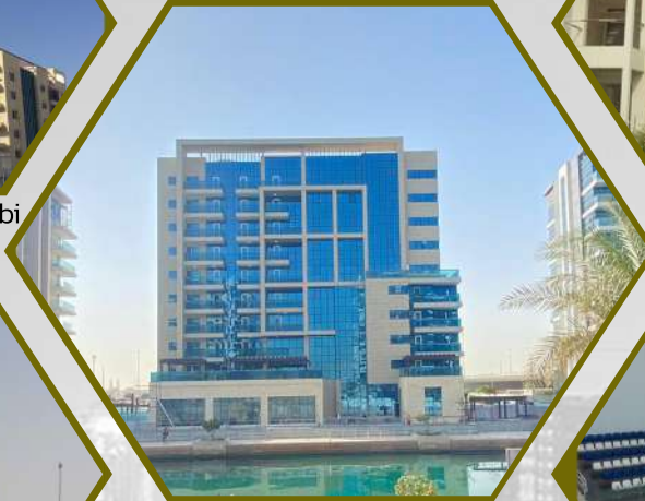
Commercial Tower G+9 - Abu Dhabi
