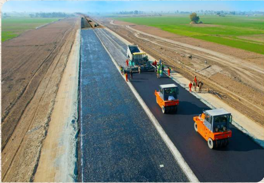
Gujranwala - Lahore Sialkot Motorway Dual Carriageway
