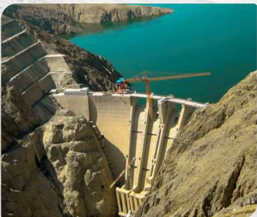
Gomal Zam Dam - South Waziristan
