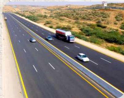
Karachi - Hyderabad Motorway (M-9)
