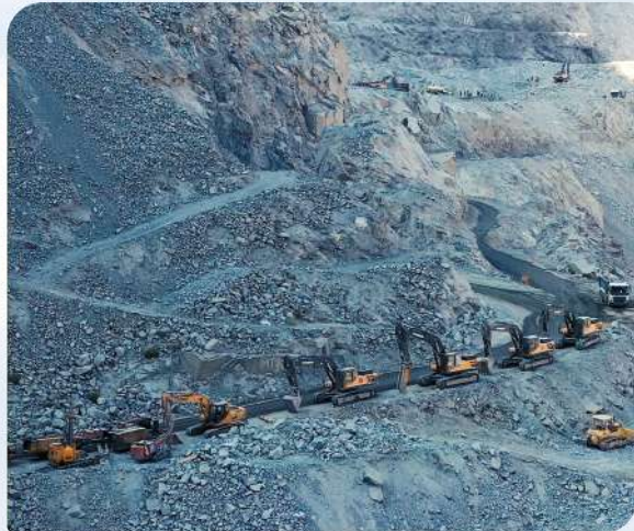
DIAMER BASHA DAM
